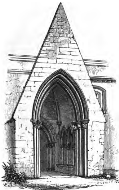
110. Barnack, Northamptonshire, c. 1250.
